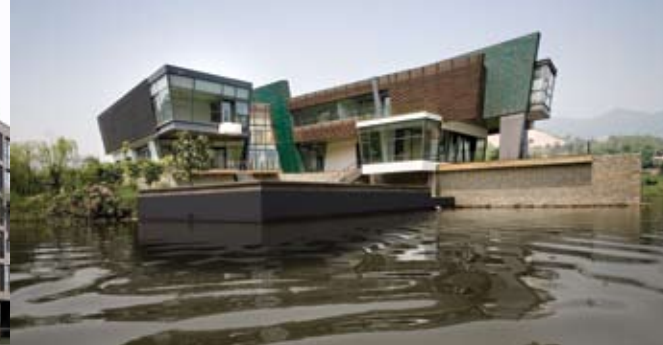
Chongqing Jade Lake residence
