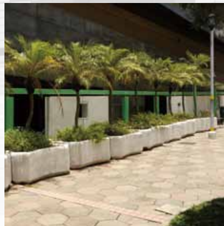
Fence Wall Before Renovation
