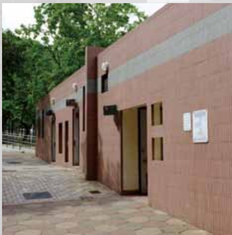
Toilet Block Before Renovation
